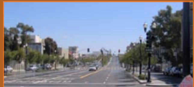
Multiway boulevards provide tree-lined streets with separate realms for through-traffic and for slow-paced vehicular-pedestrian movements.
