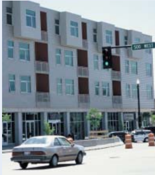
THE BRIDGE PROJECTS
