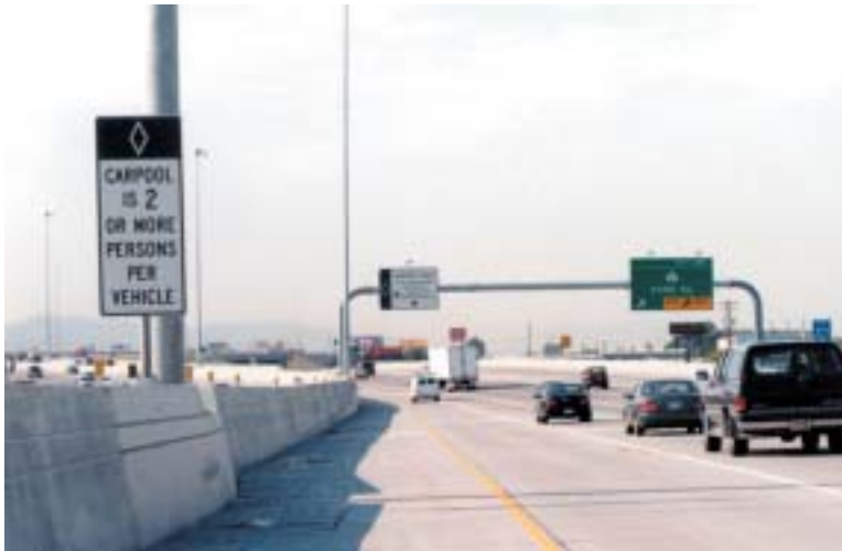
HOV LANE ON I-15, SALT LAKE CITY, UT
