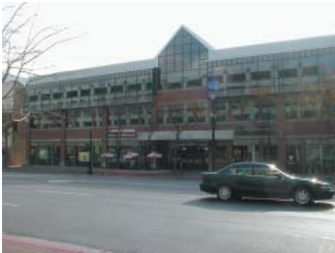
THIS WASATCH FRONT BUILDING SUCCESSFULLY ILLUSTRATES TRANSPARENCY AND INTERACTION BETWEEN THE PUBLIC AND PRIVATE REALMS
