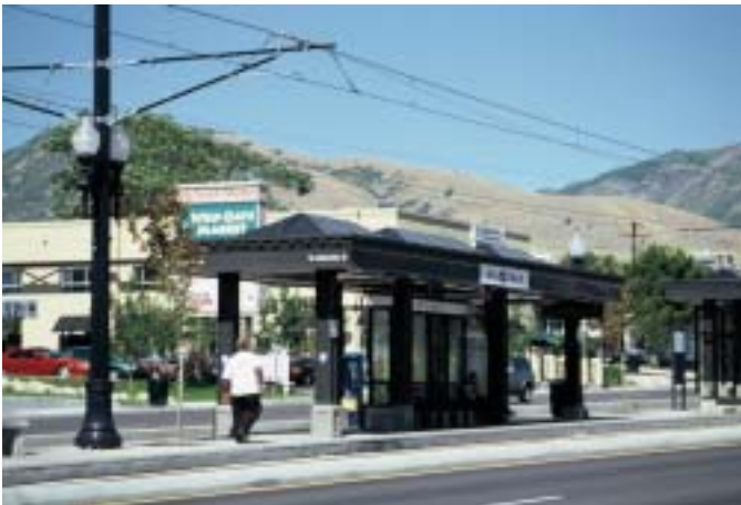
600 EAST LIGHT RAIL STATION, SALT LAKE CITY
